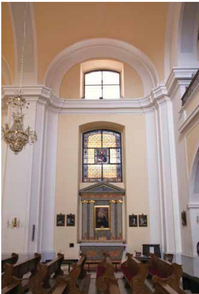
Travej kupolastog svoda u brodu (foto: M. Drmić) Bay covered by the domical vault in the nave
