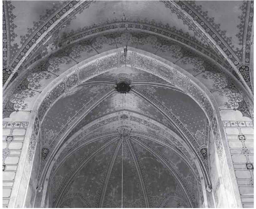
Macinec, oslikani križno-rebrasti svod Macinec, painted cross-rib vaulting
